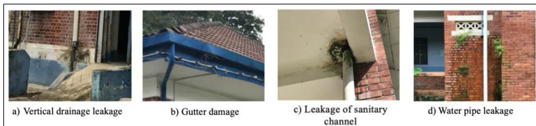
**Figure 4.** Types of Leakage and Piping Drainage Problems in the Heritage Buildings of PULAPOL Kuala Lumpur
