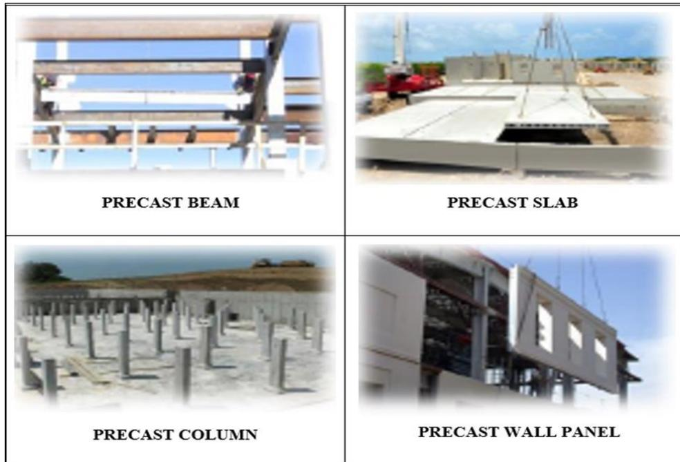
**Figure 2.** Precast Building System (CIDB, 2013)
