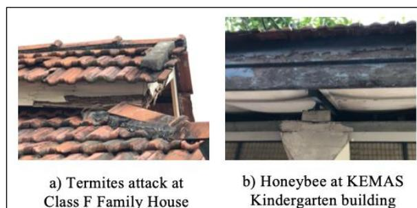
**Figure 9.** Types of Insect and Pest Attack in the Heritage Building of PULAPOL Kuala Lumpur
